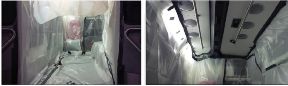
Figure 4. UNMC draping technique using 6-mil impermeable plastic.
